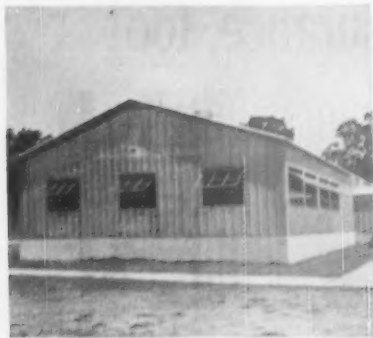
Butler die-formed steel makes a tailored finish. Note neat eaves and roof ridge, mitered joints where walls meet roof.
